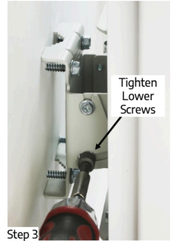
Figure 6: Elevation Bracket Installation (Wall Mount)
